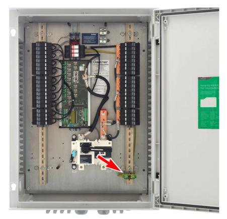
Fig. 3-13 DC Combiner Box for 20 PV strings; the ground terminal is identified.
